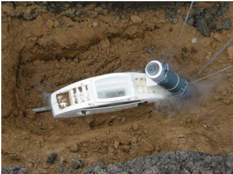
Alternatively, the length of string provided can be used to lower and tip the applicator flask. This enables use of the Cold Clamp system in confined spaces, without personnel having to enter the pit once liquid nitrogen has been poured. See the guide on the side of the flask for a convenient method of attaching and detaching the string.
